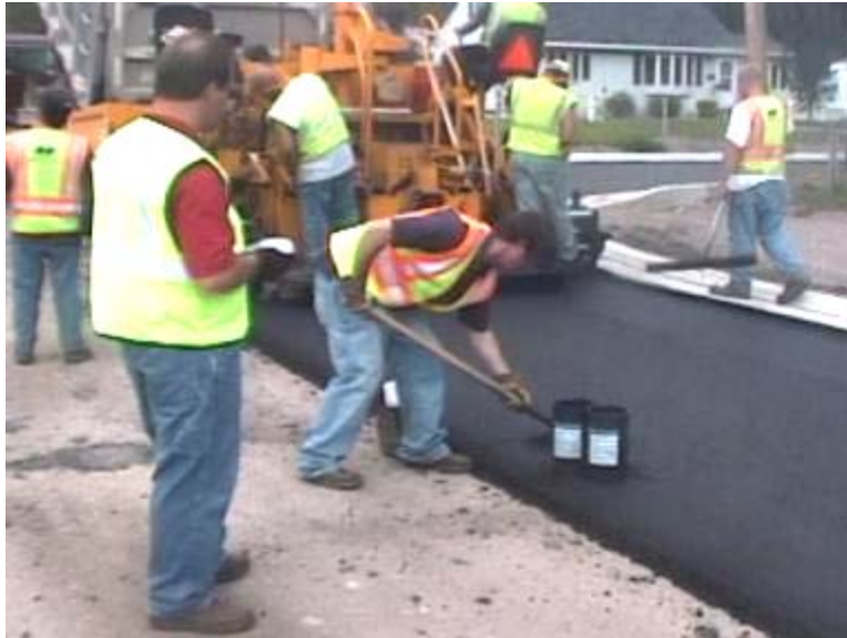
Picture 19 - HMA Sampling Behind the Paver
